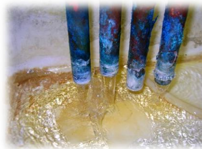
Figure 8: discharge pipes from mains-to-drain cooling in the Physical Chemistry Building
